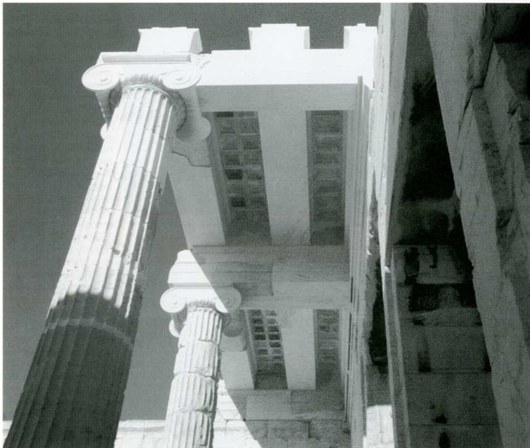
The restored ceiling of the West Hall of the Propylaea. Photo T. Tanoulas, December 2008
