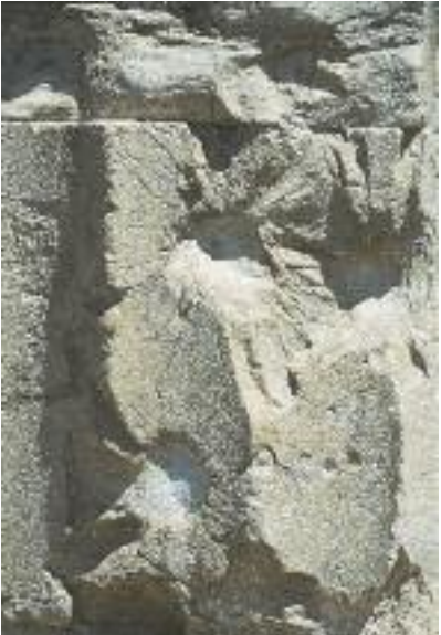
Traces from cannon balls and bullets on a column on the west side of the Parthenon.
