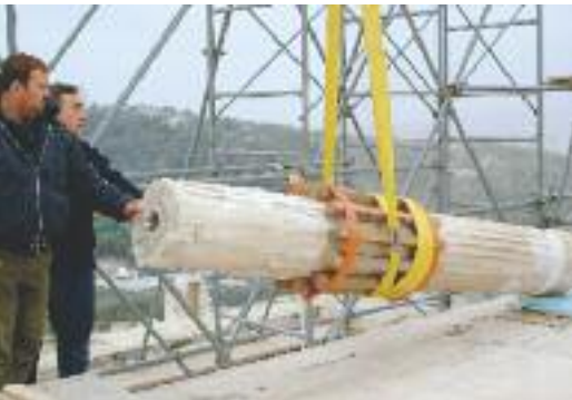
Dismantling the capital and moving the shaft of a monolithic column from the temple of Athena Nike.
