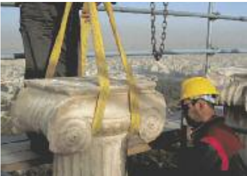
Dismantling the capital and moving the shaft of a monolithic column from the temple of Athena Nike.
