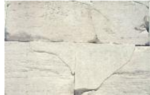
Reversibility. Using appropriate technical methods fragmented ancient marble and supplements are joined together without necessitating any chiselling.
