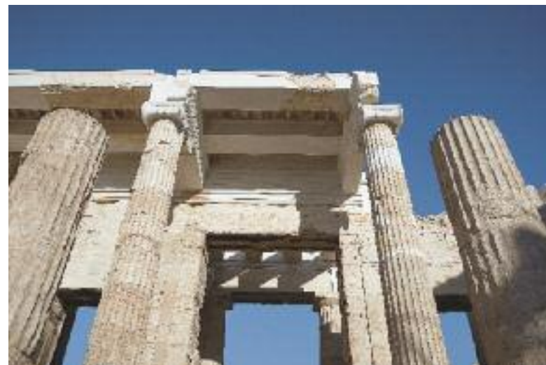
Section of the Propylaia's ceiling after the restoration.
