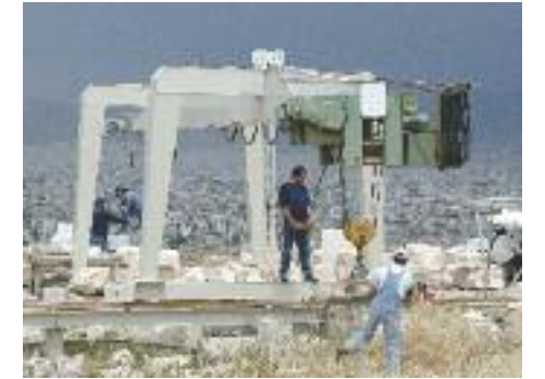
Bridge crane on ground level rails at the Propylaia work-site.
