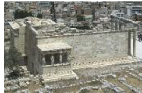
The south side of the Erechtheion. Correction of earlier misplacement of wall blocks, with the addition of new marble where necessary.
