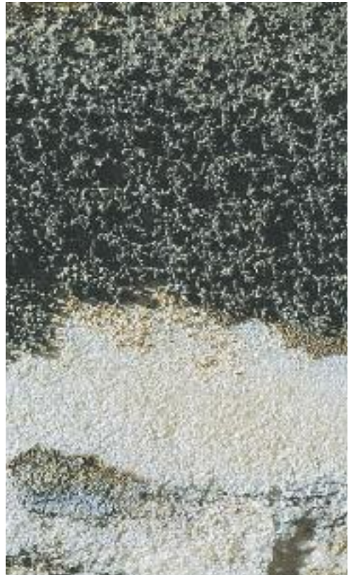
Various deposits, a result of atmospheric pollution. Marble crystals that have lost their cohesion and form a darkened crust due to soot and dust can be discerned.
