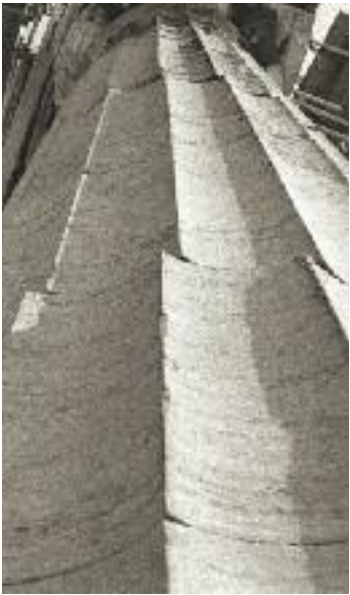
Displacement of the drums of a Parthenon column due to an earthquake.
