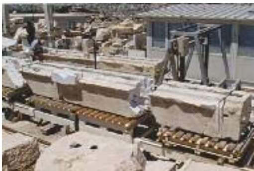
Joining together of fragments of a beam from the Propylaia's east stoa. (T.T.)
