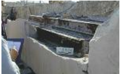
Marble cracks due to the swelling of iron elements. (YSMA Archive)
