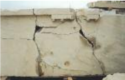
Marble cracks due to the swelling of iron elements. (YSMA Archive)
