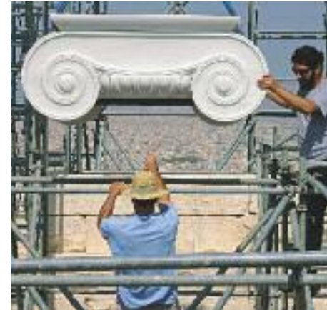
Resetting of one of the new Ionic capitals in the central hall of the Propylaia.
