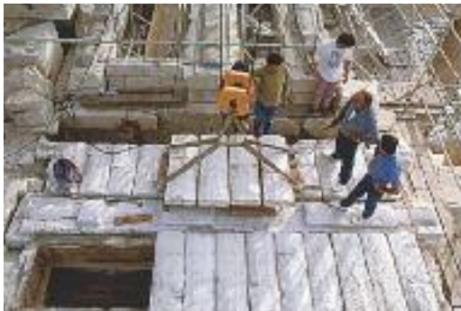
Dismantling of coffered slabs from the roof of the Propylaia's central building. (T.T.)
