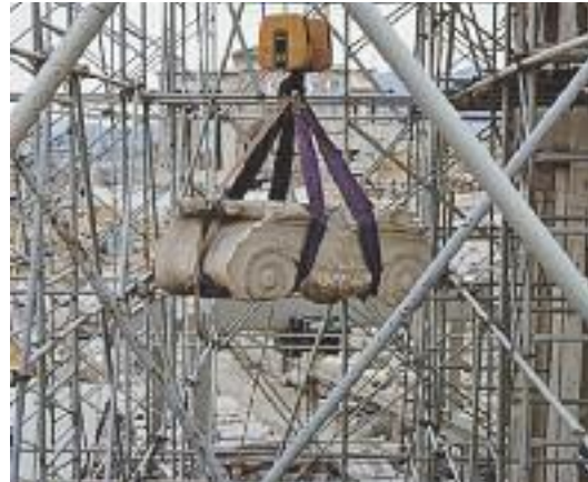
Dismantling of an Ionic capital from the central hall.
