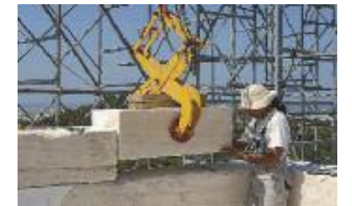
Suspension cramps for architectural members.
