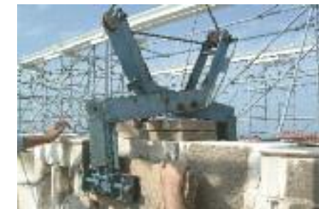
Suspension cramps for architectural members.
