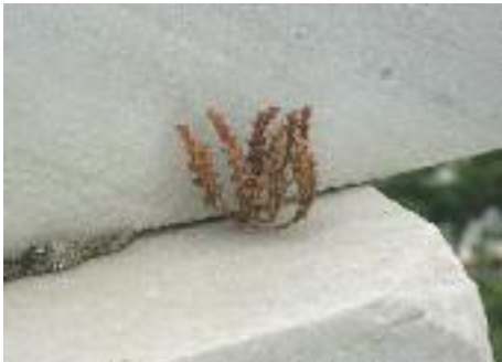
Expansion of cracks due to parasitic vegetation.
