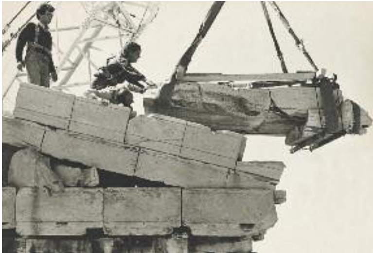
Dismantling the Parthenon's northeast sima with one of the lion-head pseudo-spouts.
