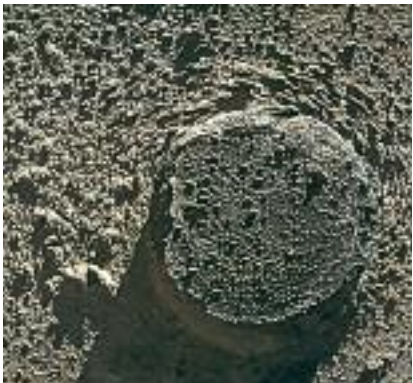
Various deposits, a result of atmospheric pollution. Marble crystals that have lost their cohesion and form a darkened crust due to soot and dust can be discerned.
