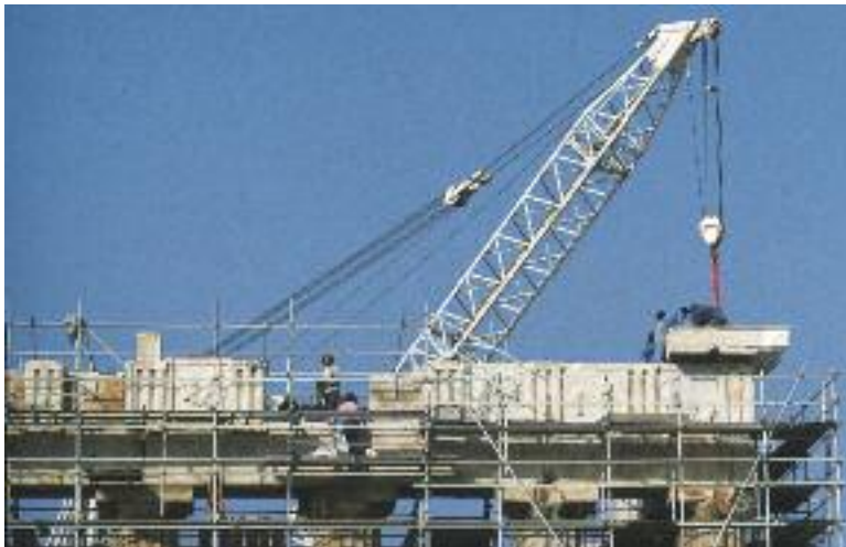
Resetting the cornice of the Parthenon's east side.
