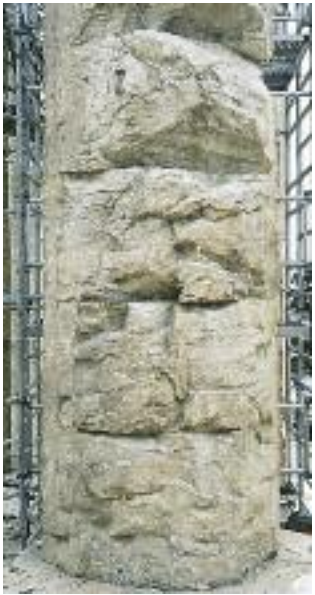
Thermal fracture to a column from the pronaos of the Parthenon.
