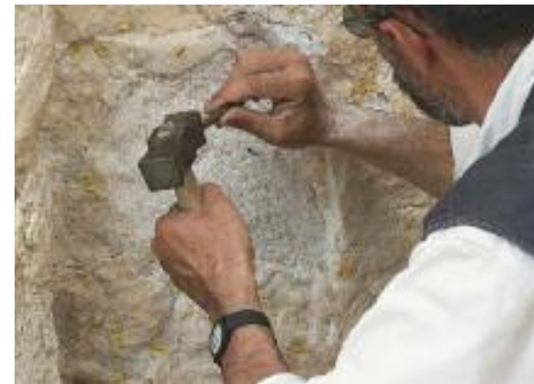
Mechanical cleaning of a marble surface.
