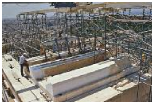
Resetting a beam from the Propylaia's east stoa. (T.T.)
