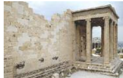
The north side of the Erechtheion. Limitation of the addition of new marble to the absolutely necessary.
