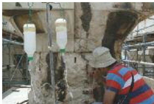
Process of joining internal cracks. Tube system in a column of the Parthenon opisthonaos, for injections of stabilising compound.
