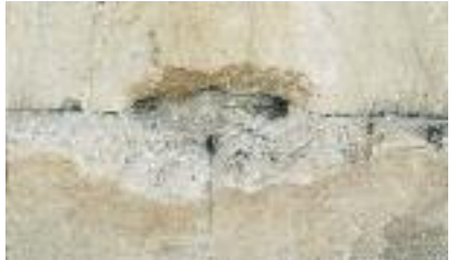
Marks from the forcible extraction of lead for the production of bullets.
