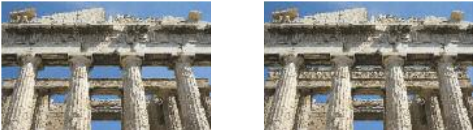
The west façade of the Parthenon during the intervention and after completion of the restoration. Approximately 130 architectural members from the opisthonaos were dismantled, repaired and returned to their positions. All the frieze blocks were removed and transferred to the Museum, while copies in artificial stone were put in their place on the monument.
