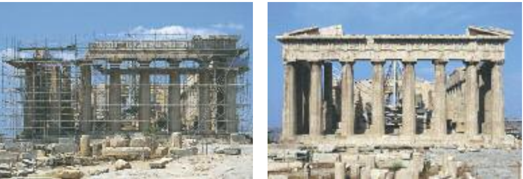
The east façade of the Parthenon during and after completion of restoration. On the east side 160 architectural members were dismantled. They underwent repairs and conservation work and were returned to their positions. All of the metopes were removed and transferred to the Museum, while on the monument they were replaced with copies of artificial stone.
