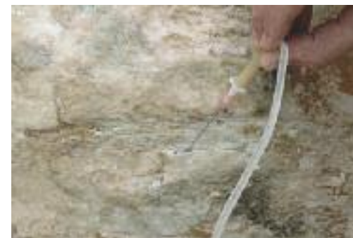
Process of joining internal cracks. Tube system in a column of the Parthenon opisthonaos, for injections of stabilising compound.
