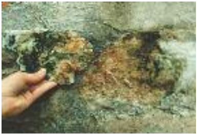
Corrosion of marble due to microorganisms.
