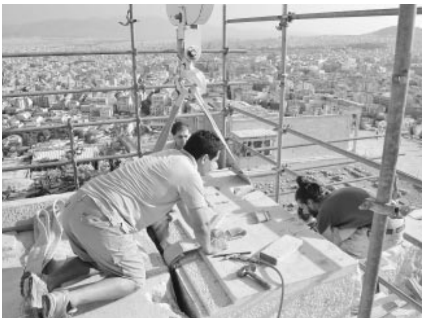
Preparations for dismantling a cornice block from the north entablature of the Parthenon. Photo V. Eleftheriou, 2011
