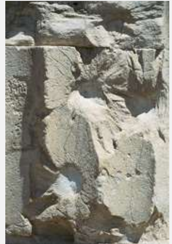
Traces from cannon balls and bullets on a column of the Parthenon
