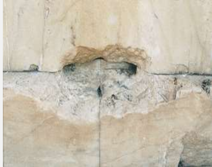
Marks from the forcible extraction of lead for the production of bullets
