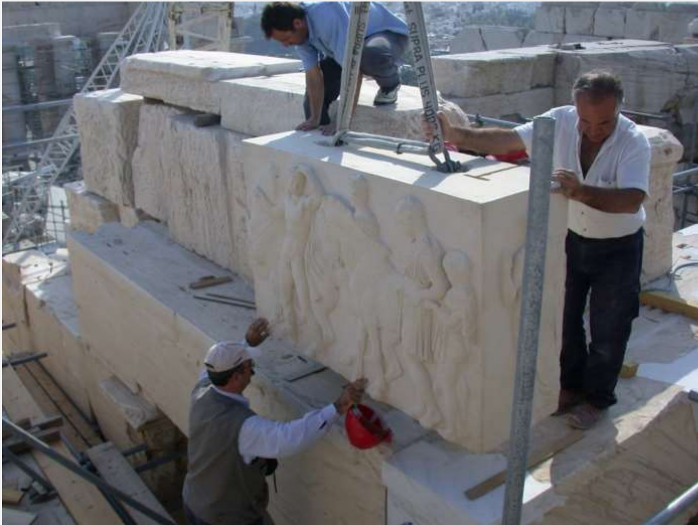
Resetting a copy in artificial stone of the west frieze in its place on the monument.
