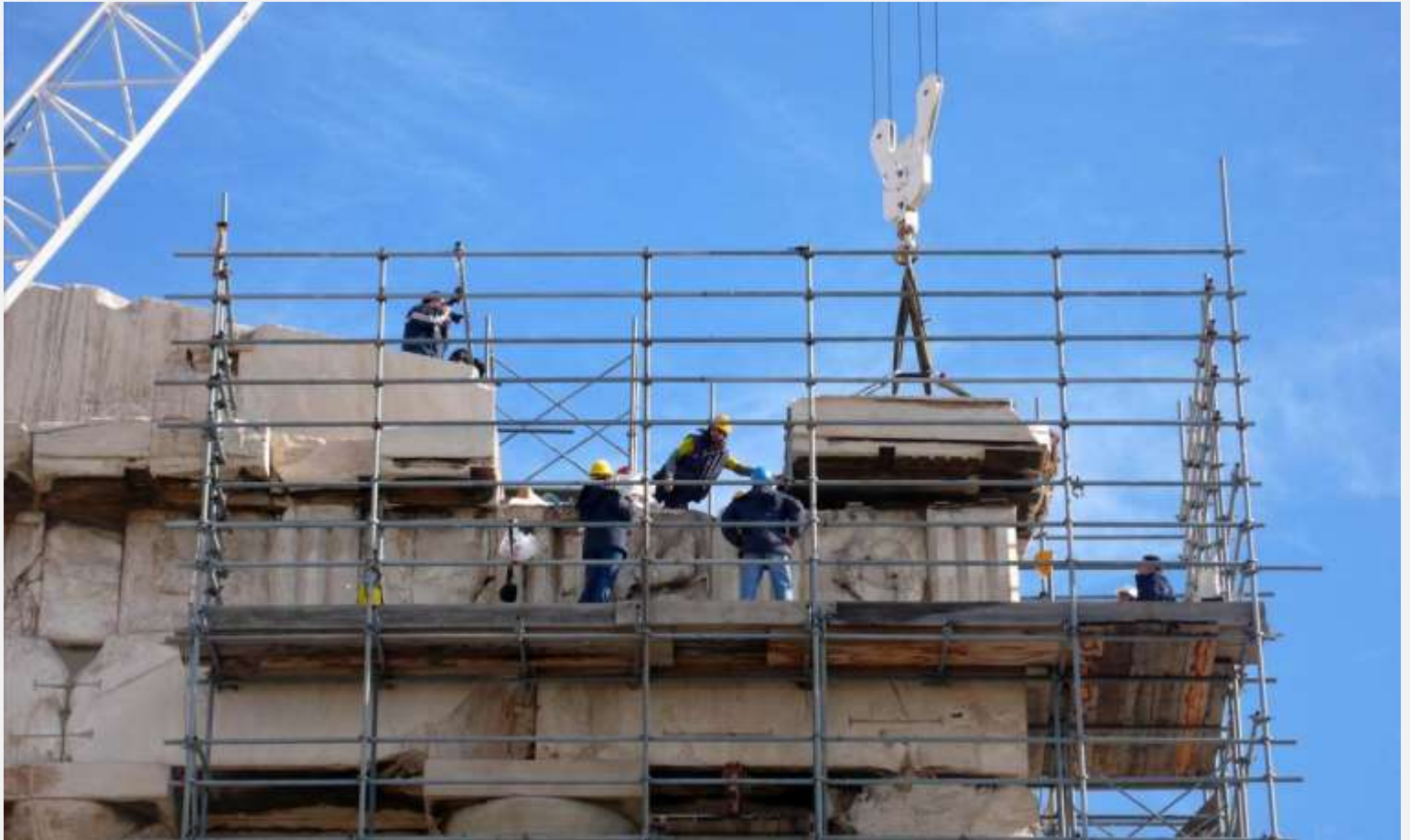
Dismantling of the SW cornice of the Parthenon.
