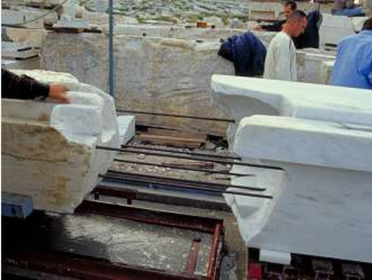
Structural restoration with titanium reinforcements
