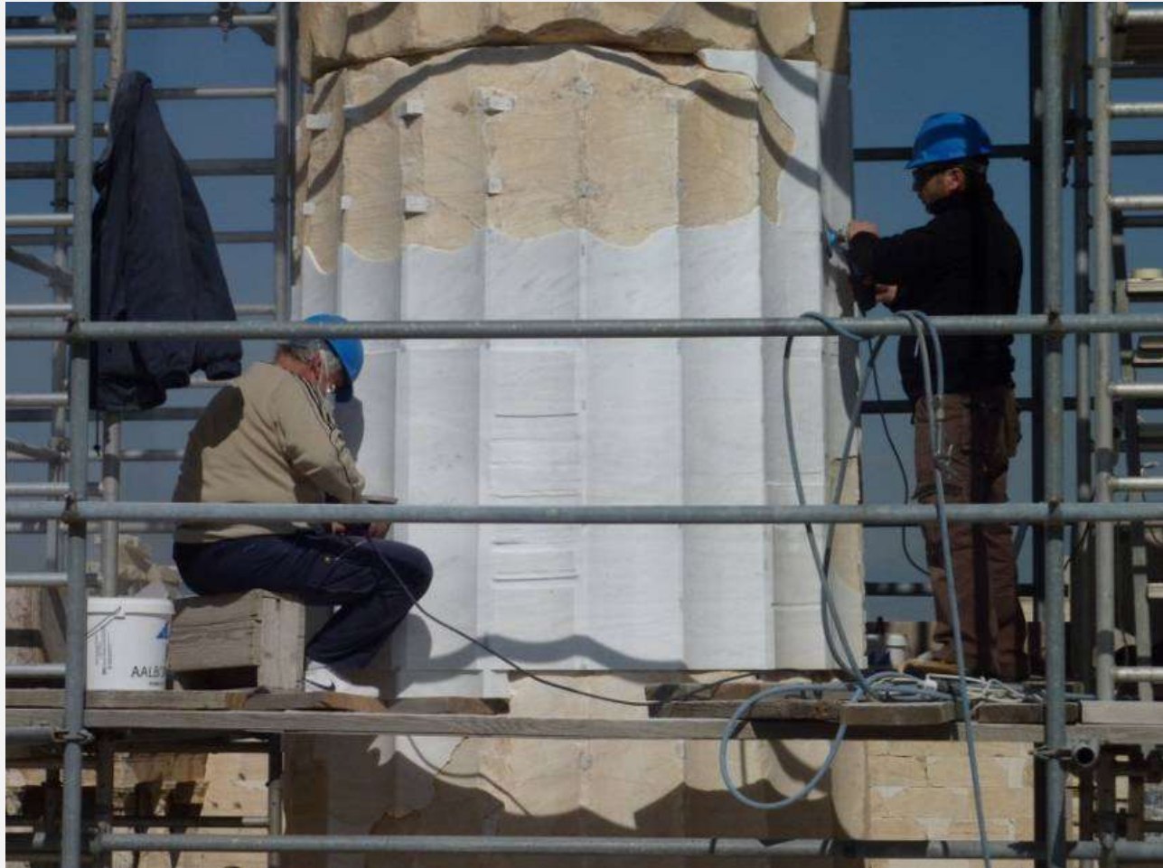
Final curving of the flutes on a column drum
