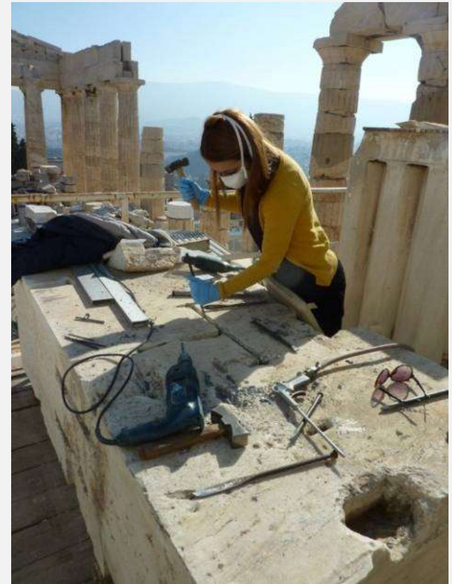
Removal of the rusted iron from older restorations.
